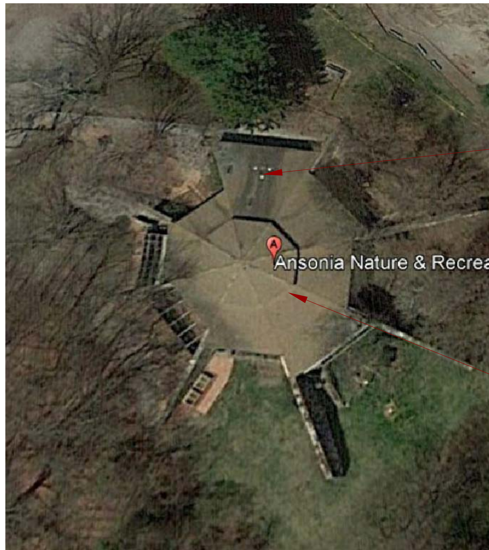
P1 AERIAL PHOTO OF ROOF
