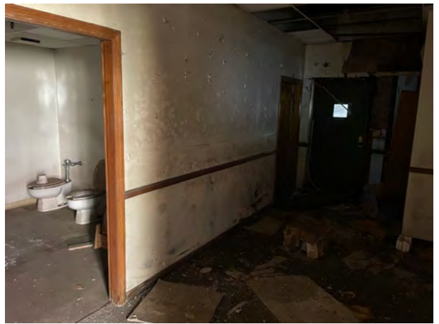
3 rd Floor Looking Into Bathrooms
