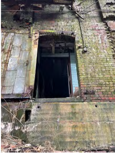
Entrance to 2 nd Floor Locker Room
