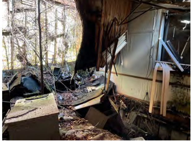
3 rd Floor North End
