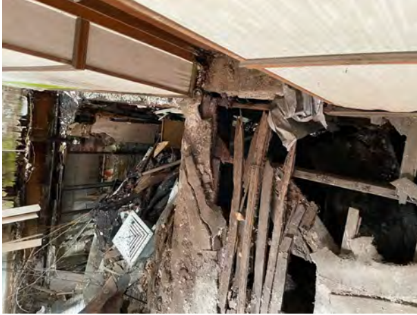
3 rd Floor North End Looking Through Floor
