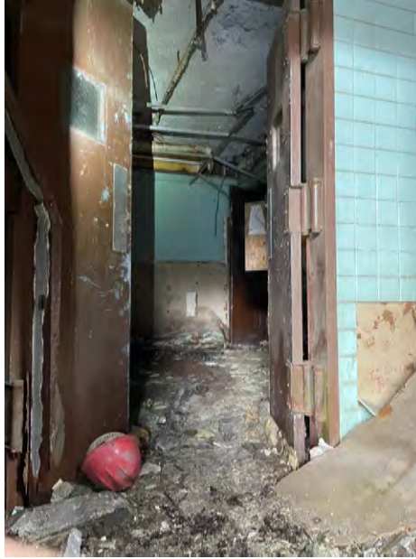
2 nd Floor Locker Room
